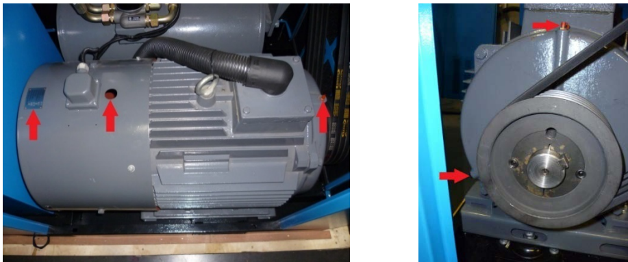
Figure 6-5 Motor Bearing Re-Greasing
