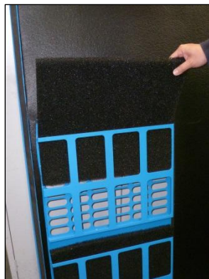
Figure 7 Air Pre-Filters Removal
