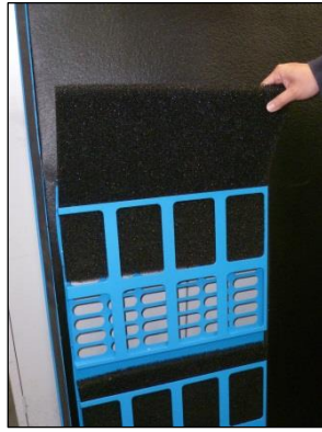
Figure 6-2 Air Pre-Filters Removal
