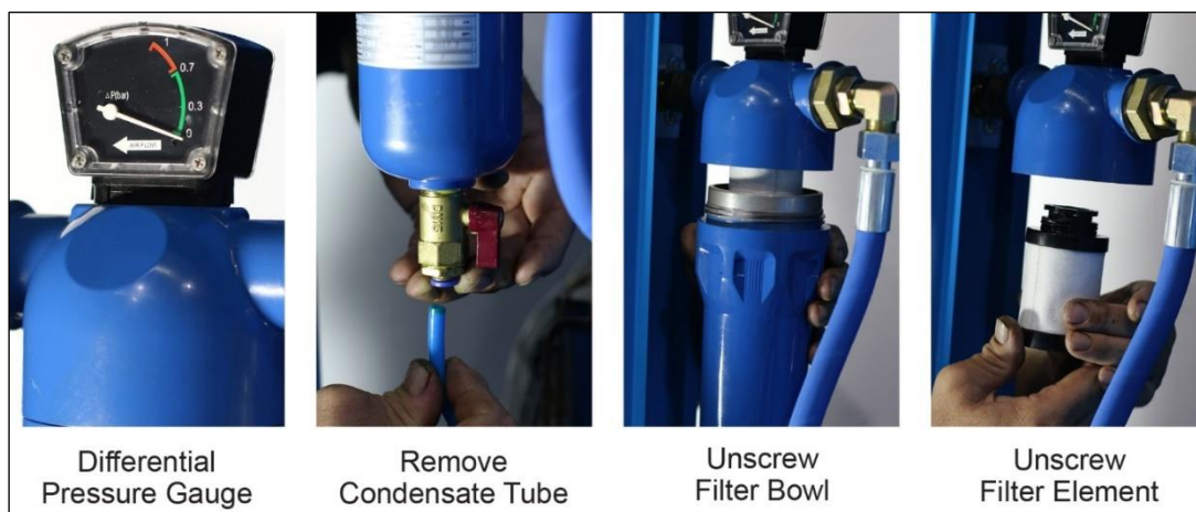
Figure 6-4 Compressed Air Filter Replacement
