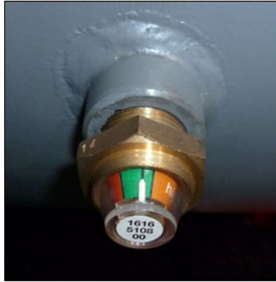
Figure 6-1 Full Oil Level Indication
