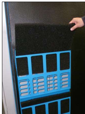
Figure 6-2 Air Pre-Filters Removal
