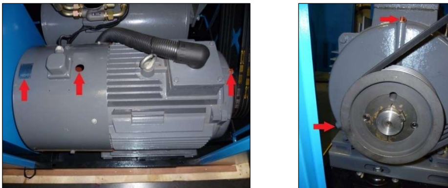
Figure 6-5 Motor Bearing Re-Greasing
